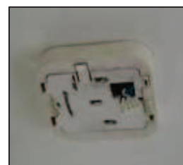
Disabled smoke alarm with the cover removed
