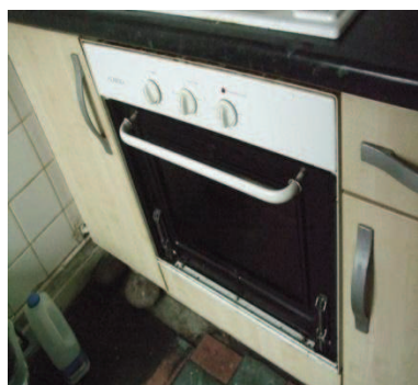
Front panel missing off oven
