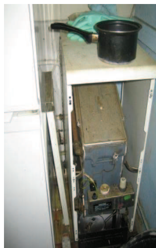
Damaged boiler with front panel missing
