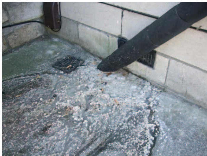
Blocked front drain
