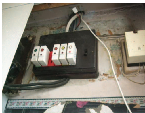
Fuse board, dated and no earthing
