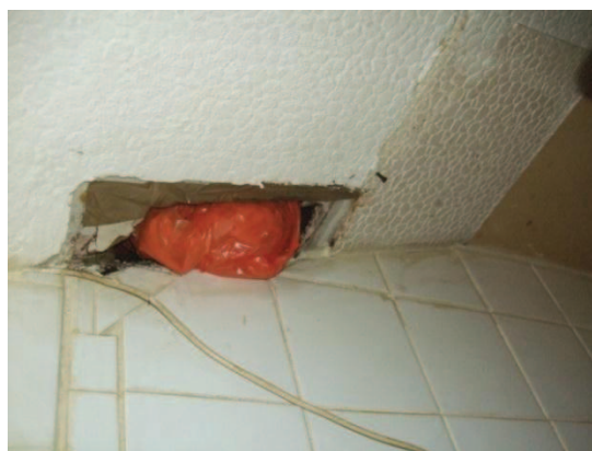
Hole in kitchen ceiling stuffed with plastic bag
